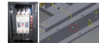
Figure 3.3 Grounding terminal
