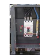
Figure 3.2. Gen-set field wiring of load cables 1 Load cables connecting terminal of Gen-set 2 Load cables can connect with gen-set through these Knock down holes 3 Grounding terminal (UL listed KDER, installation tool: 1/14" hex wrench)
